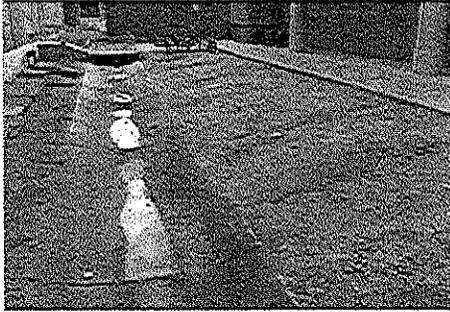
Decomposed granite migrates down on the slightest slope and makes pavements hazardous for pedestrians.
