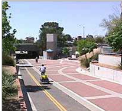
Warren Avenue underpass
