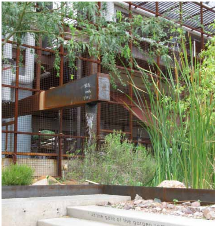
CALA building addition green wall (behind) and the multi-habitat bioswale and demonstration garden with recycled rain water (in front).
