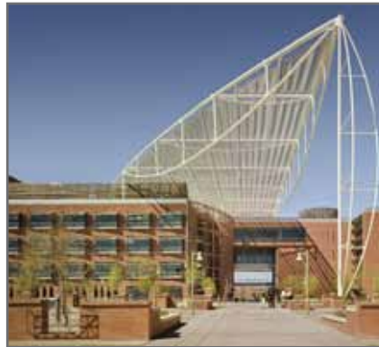
Thomas W. Keating Bioresearch Building
